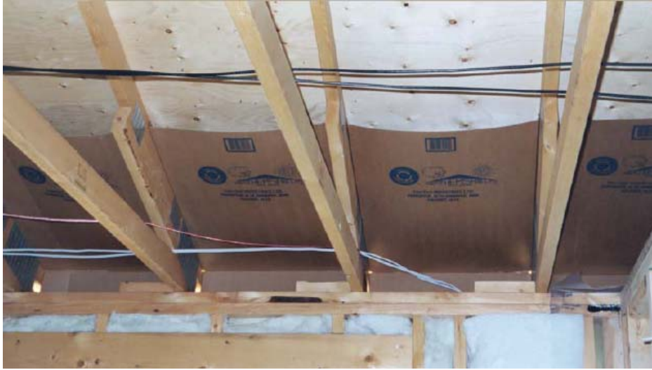
Figure 9.2 - Cardboard baffles installed to protect insulation
