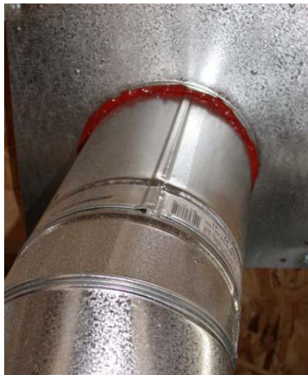
Figure 8.4 - Fire-rated caulk around a flue shaft
