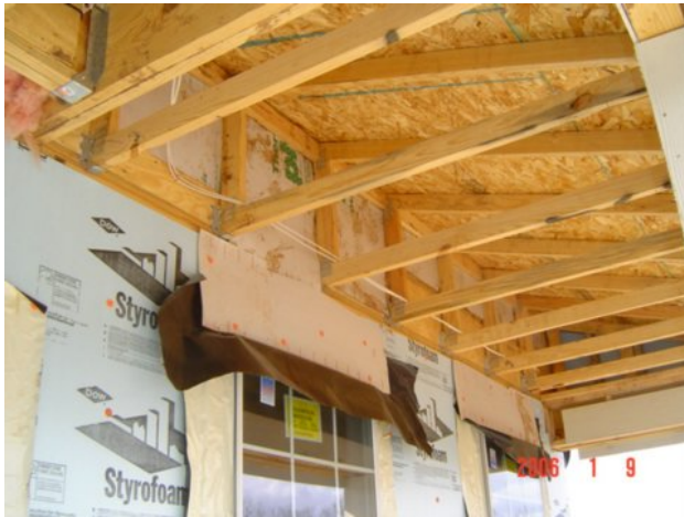
Figure 14.4 - Exterior view of blocking between porch roof and wall
