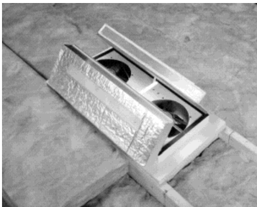
Figure 15.2 - Whole-house fan with built-in cover
