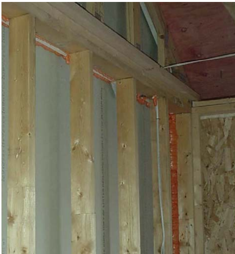
Figure 16.4 - Example of properly air sealed common wall with fire-rated caulking (in red)
