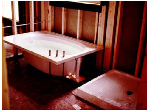
Figure 2.1 - Tub installed against exterior wall without air barrier or insulation
