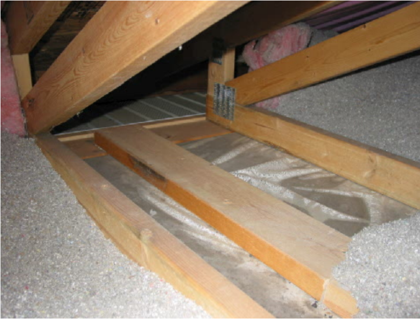
Figure 9.1 - Wind intrusion around a soffit vent
