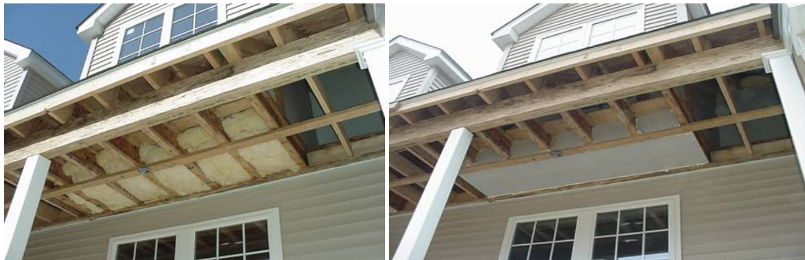
Figure 6.4 - Proper installation of insulation under a cantilevered floor
