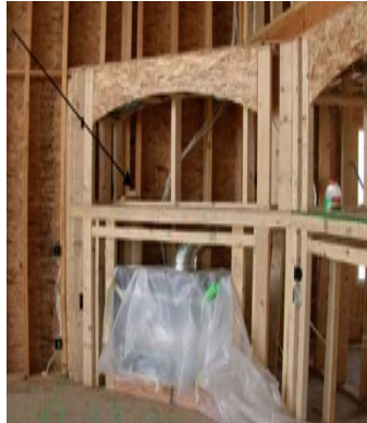
Figure 11.1 - Fireplace installed without air barrier
