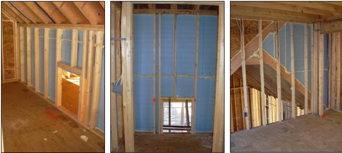
Figure 4.3 - Examples of properly blocked and air sealed attic knee walls
