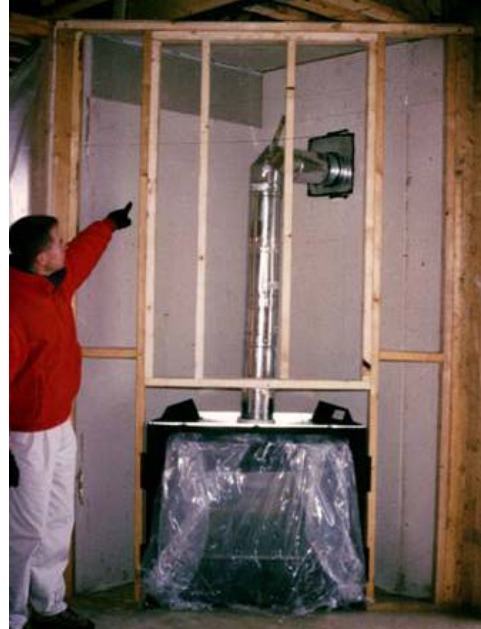
Image courtesy of Building Science Corp
