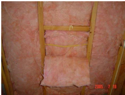
Figure 1.8 - Insulation is fit around piping and wiring
