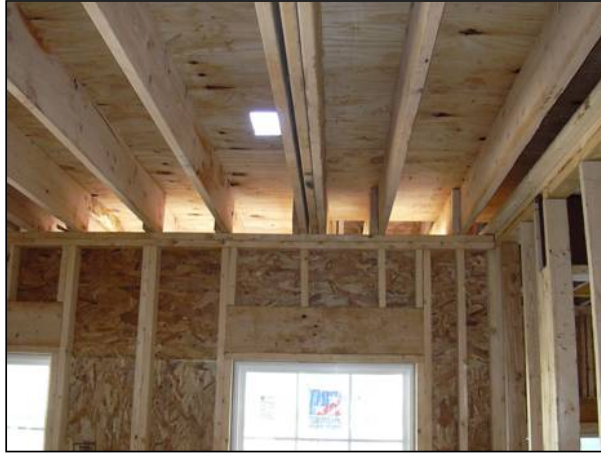
Figure 14.1 - Interior of the home is exposed to exterior air infiltration via the porch roof
