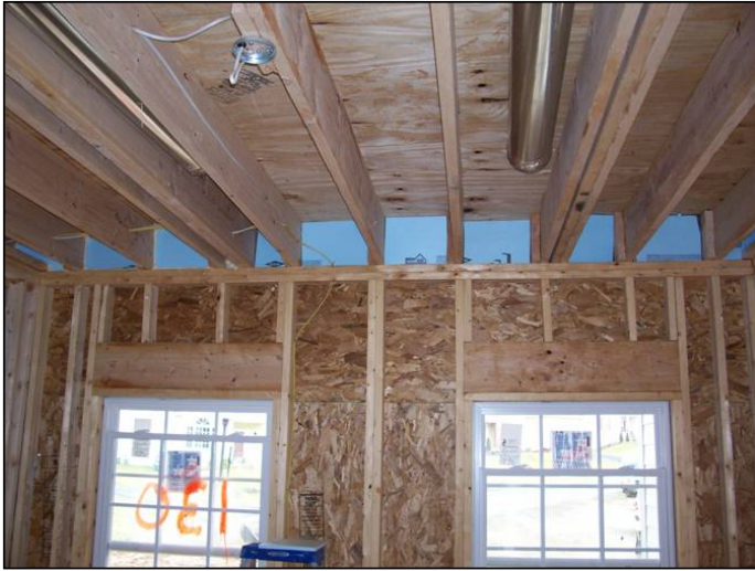
Figure 14.3 - Conditioned space separated from exterior by blue colored blocking at intersection of porch roof and wall
