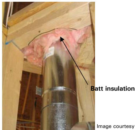
Figure 8.2 - Insulation improperly used for air sealing
