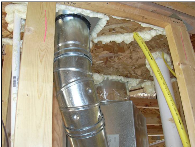
Figure 7.2 – Correct blocking and foam air sealing in a chase
