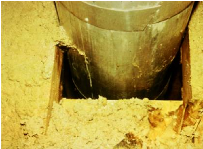
Figure 8.1 - Lack of air sealing around flue shaft
