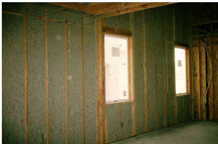
Figure 1.9 - Blown cellulose insulation
