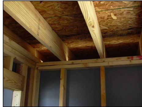
Figure 6.1 - Visible daylight indicates that there is an incomplete air barrier separating the cantilevered floor from the outside
