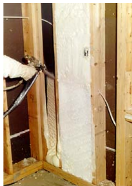
Figure 1.10 - Spray-in foam insulation
