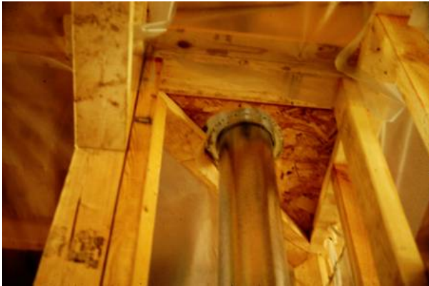
Figure 8.3 - UL-rated metal collar installed around a flue shaft
