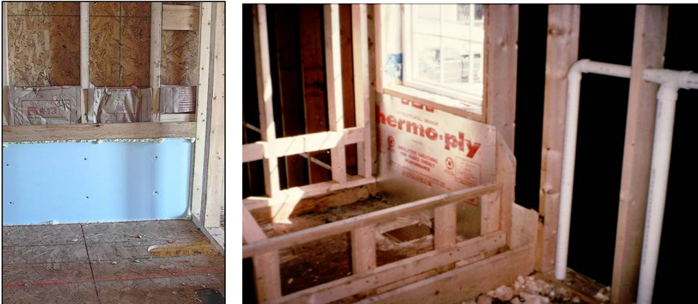
Figure 2.3 - Detail of tub installation with complete air and thermal barriers
