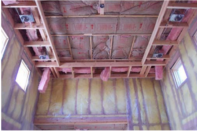
Figure 10.1 - Improperly installed insulation over a dropped ceiling
