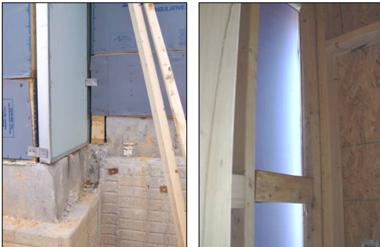
Figure 16.2 - Poorly sealed common wall
