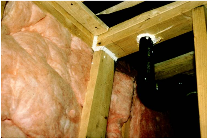
Figure 7.1 – Correct caulking around piping penetration
