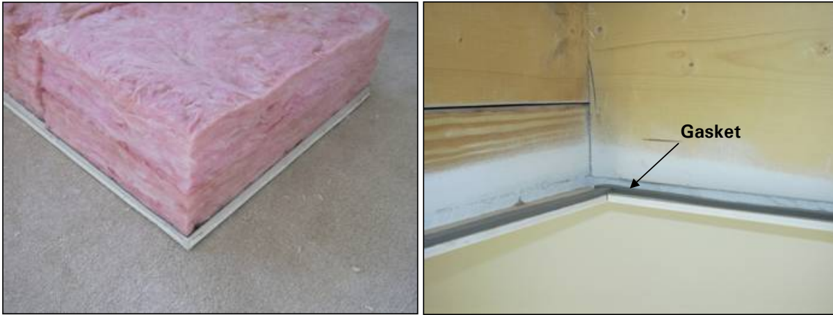
Figure 5.3 - Example of properly insulated attic hatch
